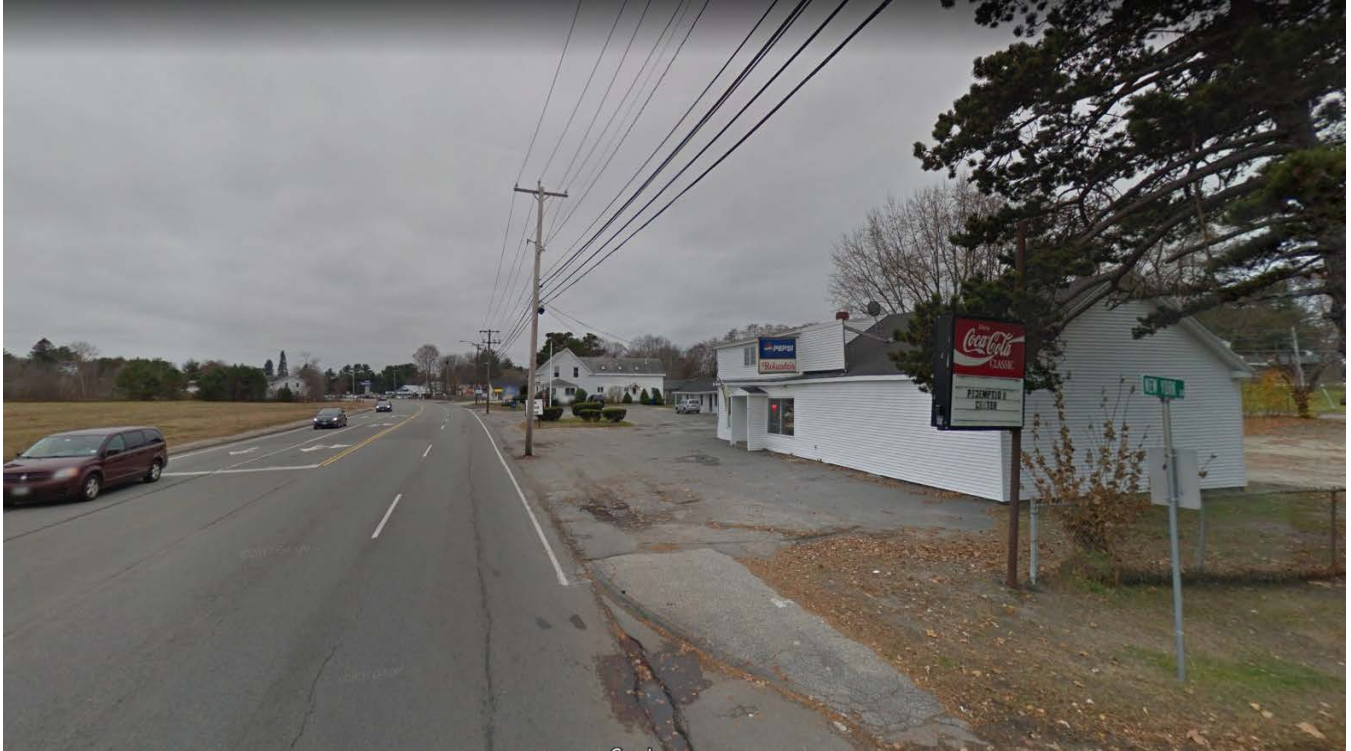
Curb Cut PRIOR to road construction
