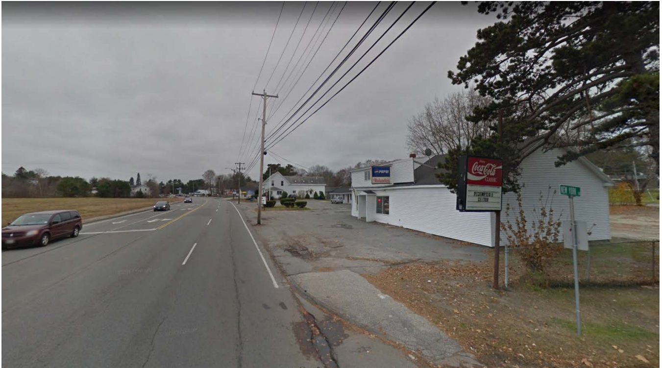
Curb Cut PRIOR to road construction
